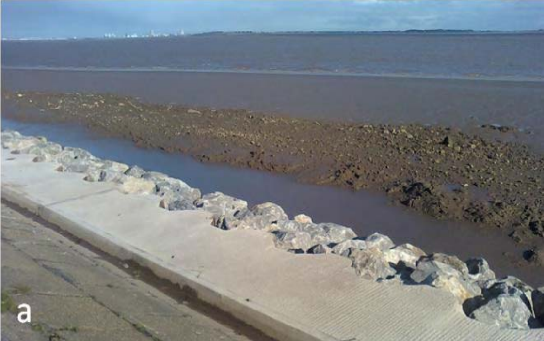
Figure 10. Exposed gravelly mud along the Killingholme foreshore.
